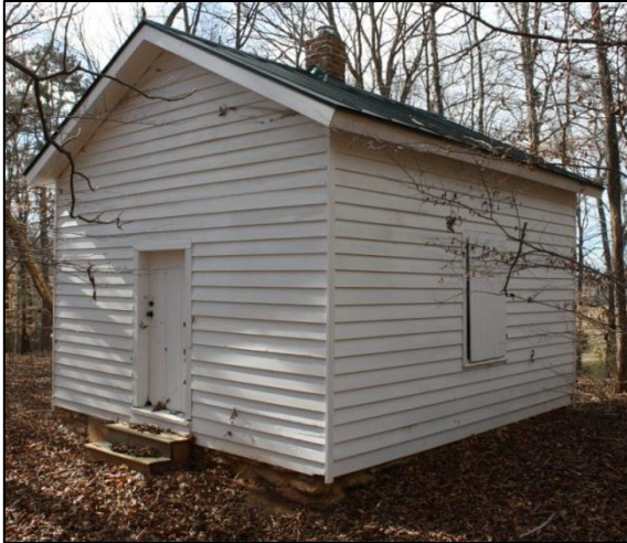
Figure 20- This School House (062-5135-0053) is said to be the first public school in Nelson County
