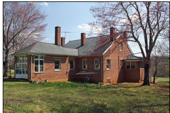
Figure 35- Arrowhead may be individually eligible for National Register listing because of its architectural character and association with Col. Wirt Robinson
