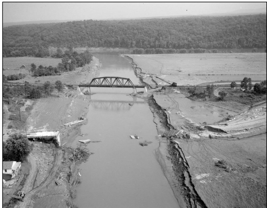
Figure 26- Hurricane Camille destroyed the Tye River road bridge at Norwood. The damaged porches of Peters Store (062-0216) can be seen in the lower left corner
