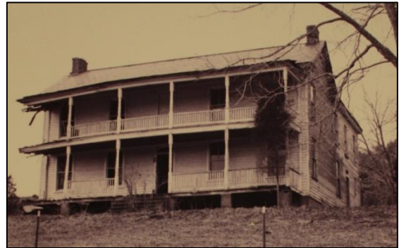
Figure 31- This dwelling (062-0232) on the west side of the Tye River is one of several that have been demolished since the last surveys were conducted in the 1990s
